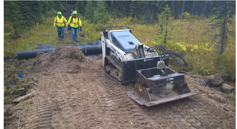
*Figure 10 Raised tread construction on the High Rockies Trail using geotextile and no ditches. Culverts are to prevent the trail from the acting like a dam and becoming saturated.*
