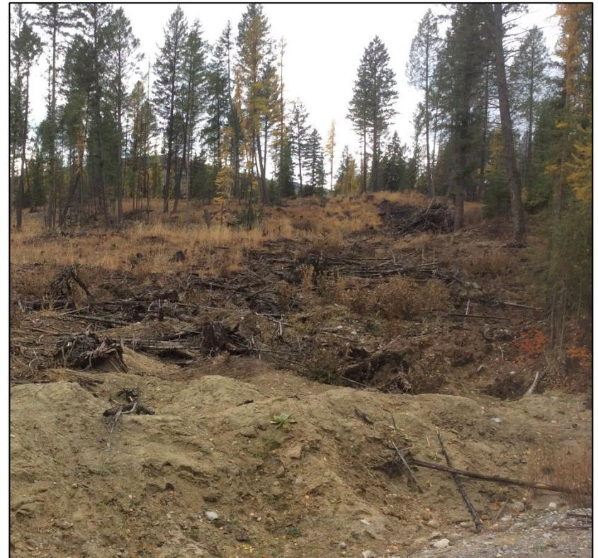
*Figure 19 Example of a decommissioned road with all signs of ditches and road shape removed. The roughened surface and debris prevent easy travel allowing vegetation to succeed.*
