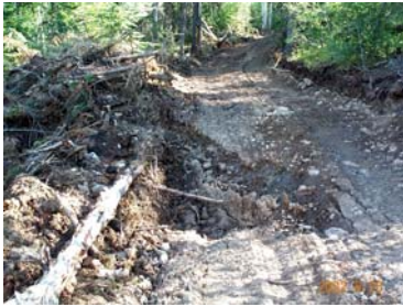
Trail washout caused by improper drainage and organic debris in the sub-grade.
