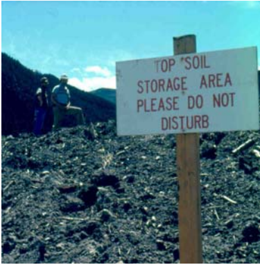
An example of soil conservation—salvaged topsoil temporarily stockpiled.
