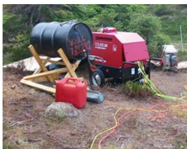
Camp generator and fuel. Note several items for improvement: the horizontal fuel drum, small drip tray, and lack of blanket material to absorb any fuel leaks
