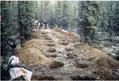
Trenching using explosives.
