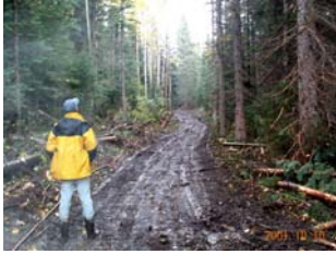
A typical access trail. Note that debris is not pushed into standing trees and is easily pulled back onto the road surface during reclamation.
