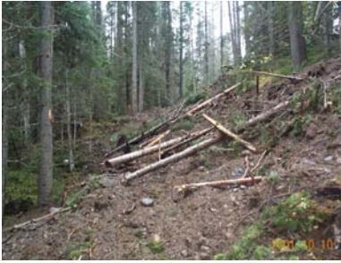
Recontoured trail on a steep slope. The site is to be seeded with grass to control erosion.
