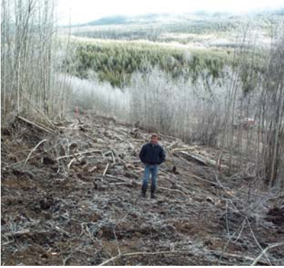
Reclaimed trench site; note the width of disturbance, which reflects the depth of overburden.
