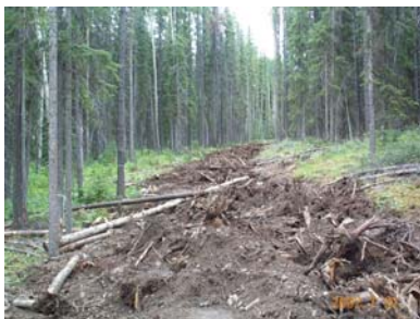
Reclaiming a road. Soil has been loosened and large debris and root balls pulled over the roughened surface.
