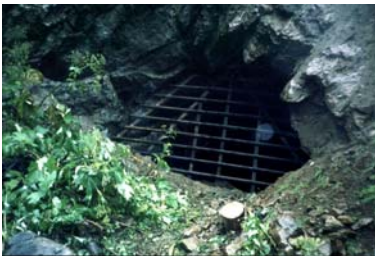
Mine opening closed with rail salvage. This allows passage for bats, permitting their colonization of old workings.
