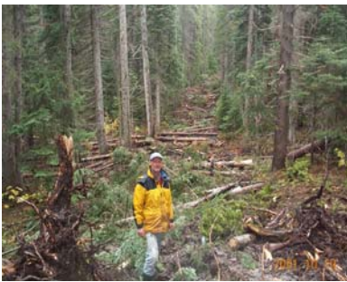
Reclaimed trail on flat terrain; nonmerchantable timber and root balls laid across to discourage use of all-terrain vehicles (ATVs).
