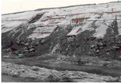
Failure of erosion-control matting.
