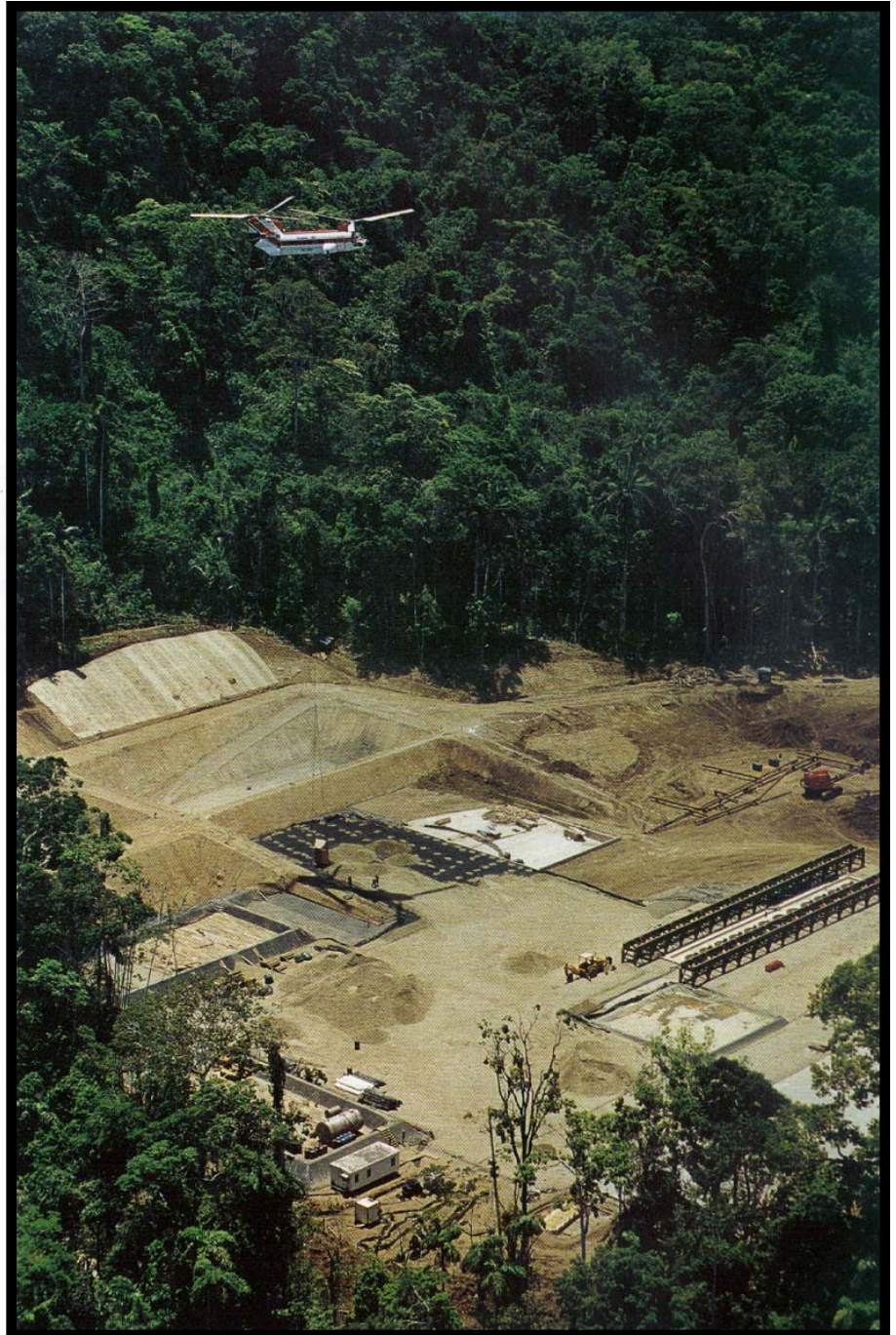
Chinook 234 slinging gravel used in Wellsite Construction
