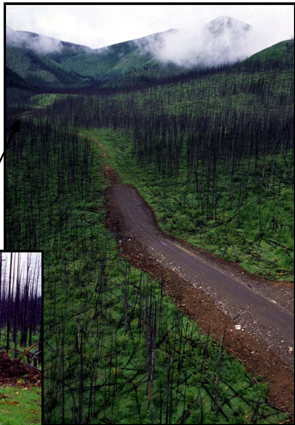
Marathon Road- end of hillside section of cut and fill
