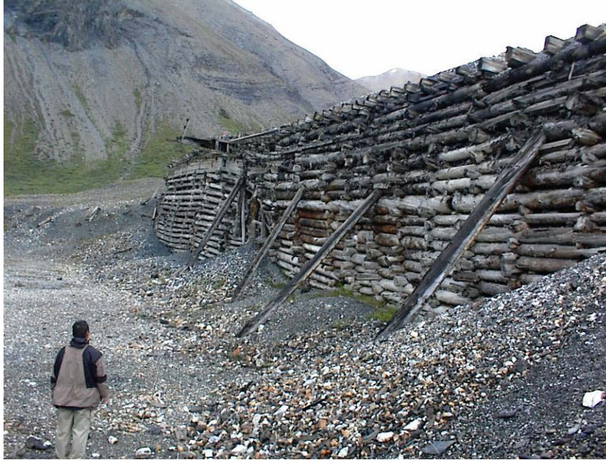
20 - Wooden Cribbed Wall At Mine Site
