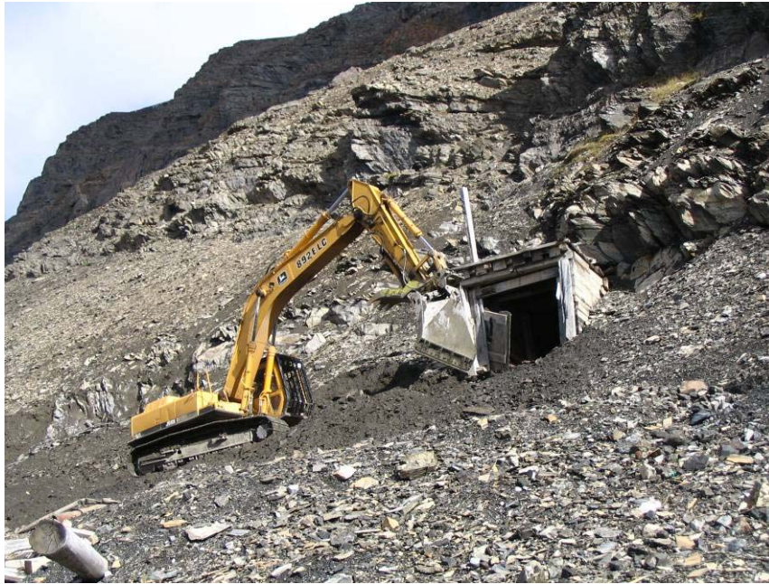
14 - Mine Adit 2 Before
