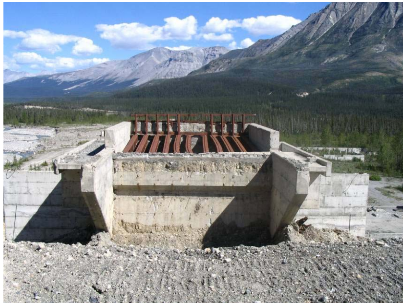
7 - Grizzly After Excavating Approach
