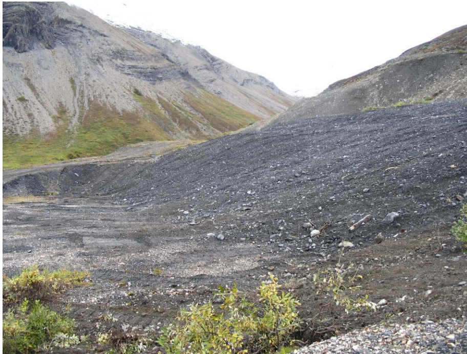
21 - Wooden Cribbed Wall Area Contoured And Covered With Soil
