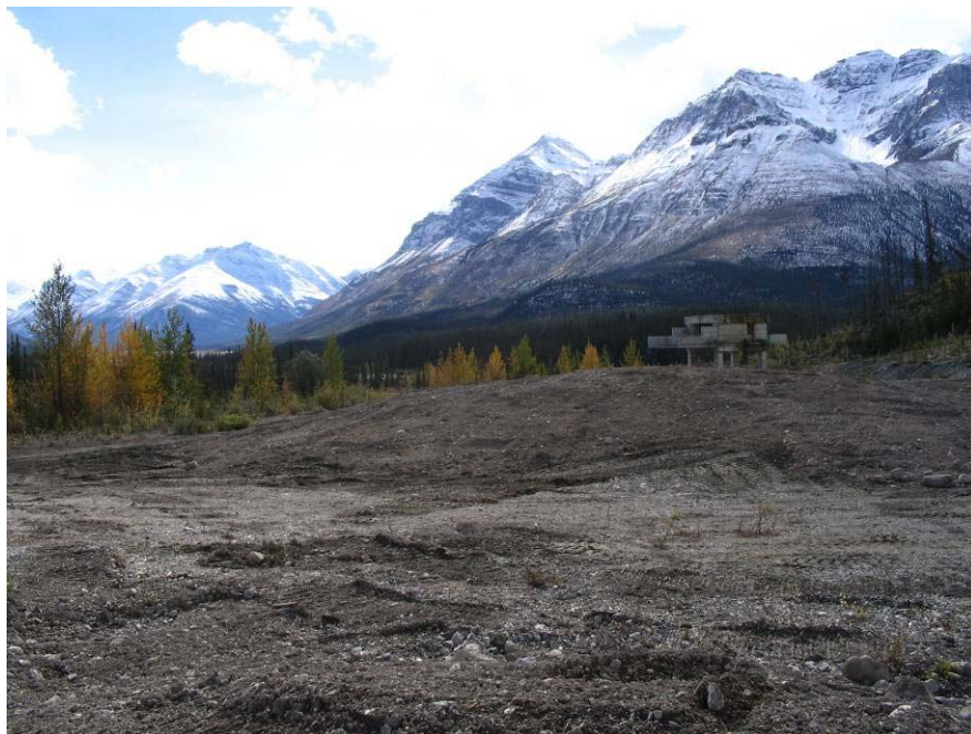
3- Mill Site After Site Preparation - looking south
