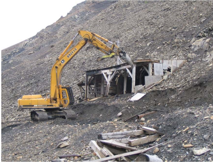
12 - Hoe Demolishing Wooden Entrance To Adit 1
