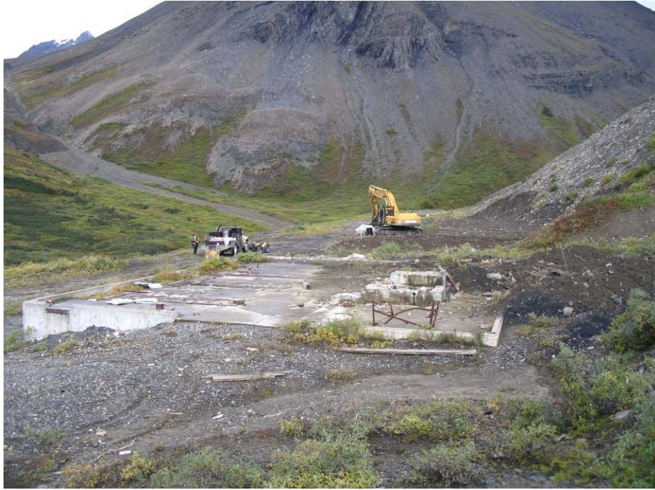
18 - Mine Building Foundations
