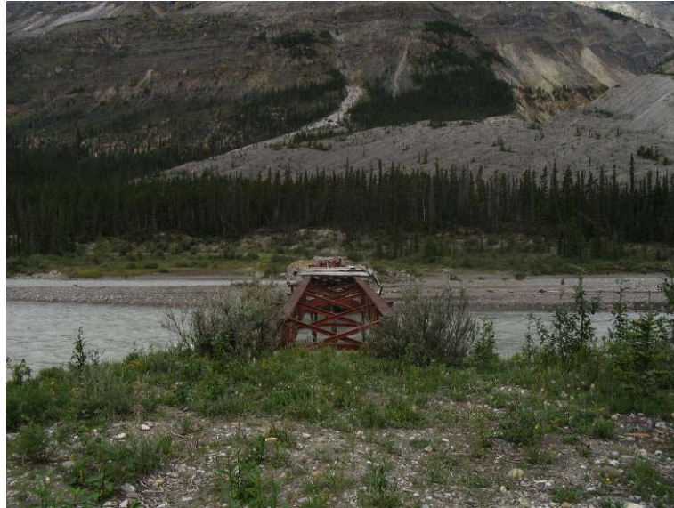
22 - East Approach To Racing River Bridge
