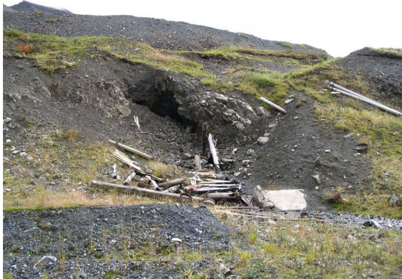
16 - Adit 3 Below Mine Building Area
