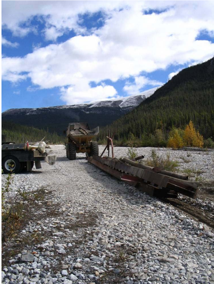
38 - Hauling Steel To Landfill Above Racing River Flood Plain
