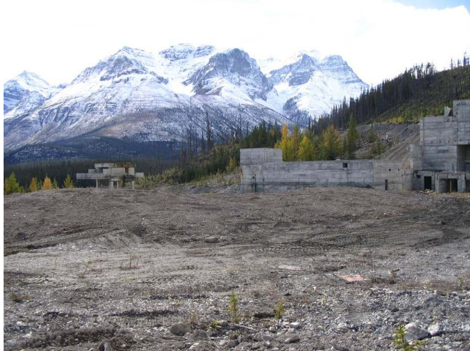
2- Mill Site After Site Preparation
