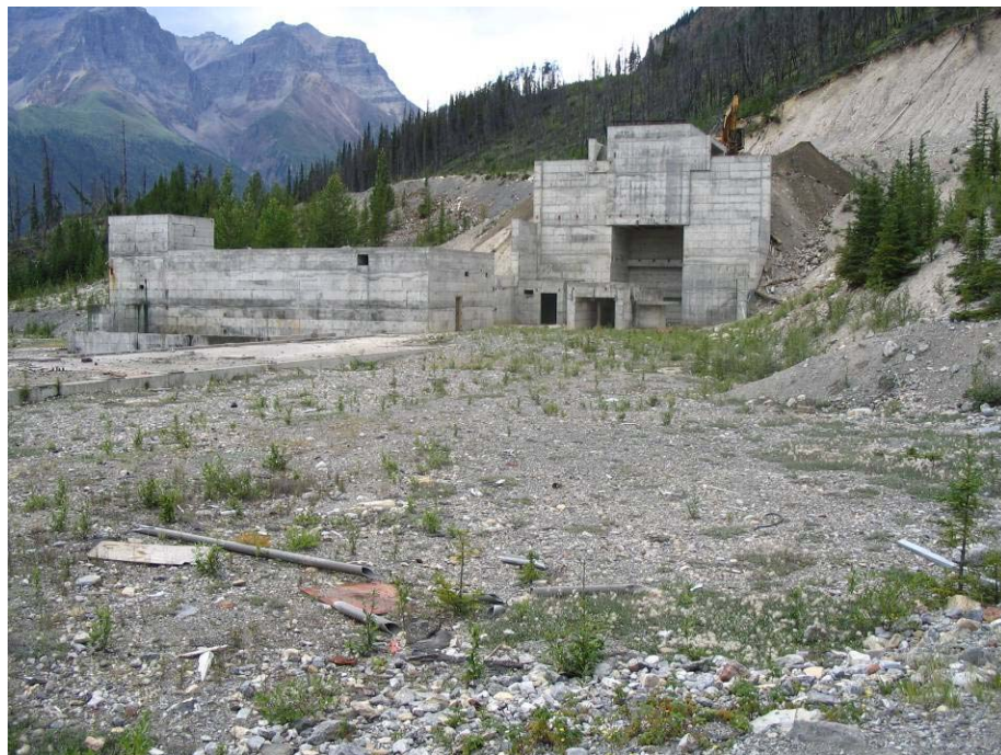
1-General Appearance of Mill Site Before Reclamation
