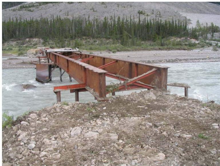
23 – East Approach To Racing River After Re-Construction
